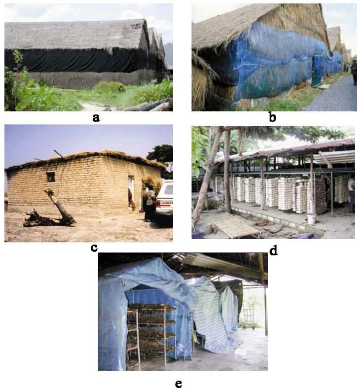
Fig. 3 (a) Thatch house with shade net, (b) Thatch house with insect net (c) Thatch house with brick walls, (d) Steel frame structure with roof, (e) Steel structure covered with tarpaulin/plastic (Source: Kwon et al. , 2004)
