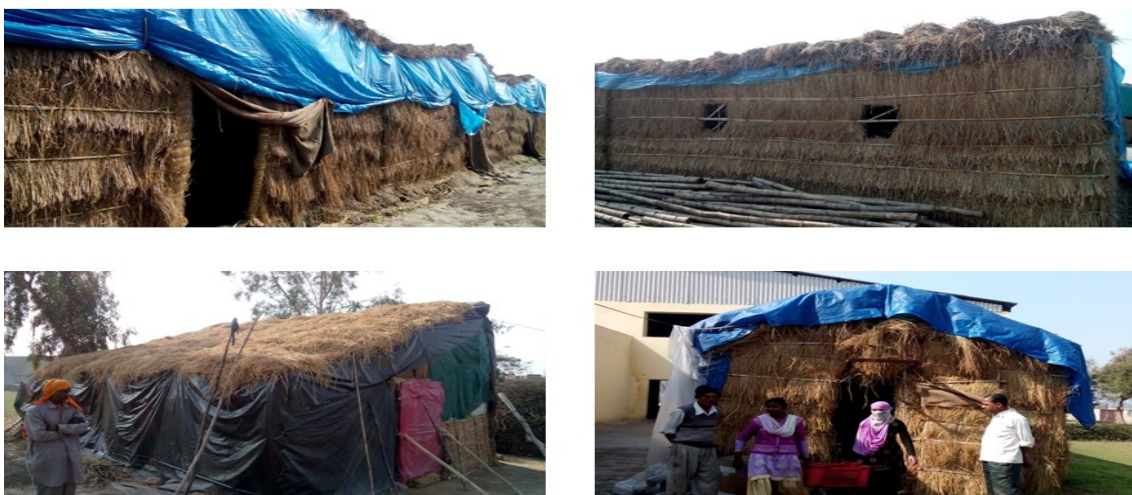
Fig.2 Structures from locally available agricultural materials in Haryana and Punjab (Photo courtesy: S. J. Kale)
