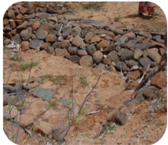
Loose boulder check dams
